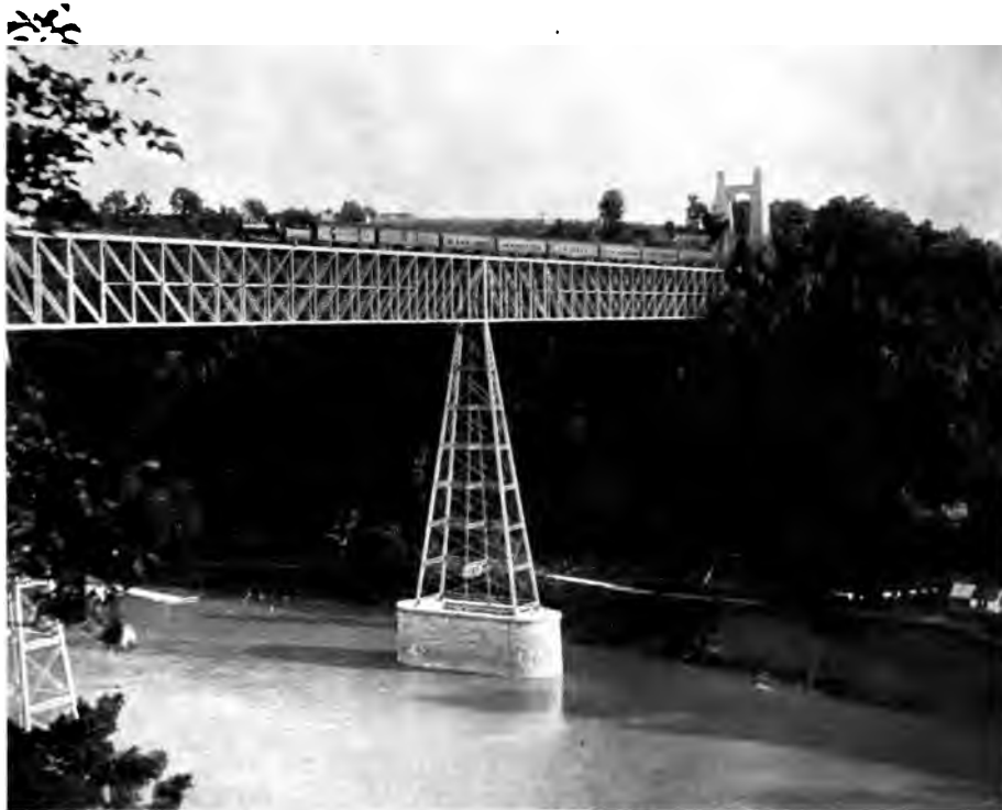
A VIEW OF HIGH BRIDGE.
